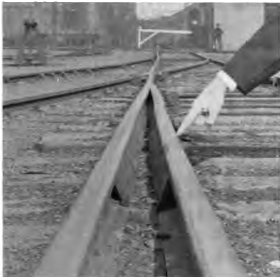
Fig. 2. Guards for Switch Points.*
